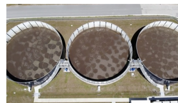
Influent flow equalization tanks 1
